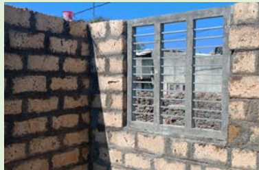
Use of locally available limestone and pre-fab window frames in rural housing projects in India.
